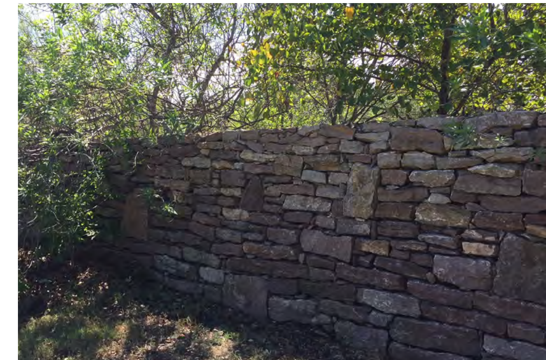
24 EXISTING HWY 71 ROCK WALL
